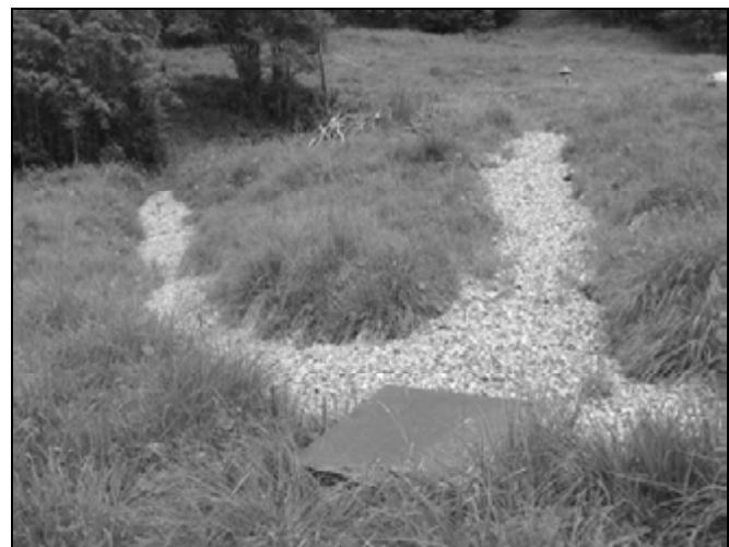
**Fig. 4. Enclosing structures: Drainage system to stabilise the sliding layers of the slope/**
