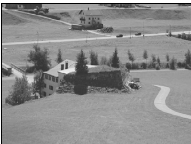
**Fig. 5. New building and upgrade: Splitting wedge for splitting and deflecting mass movements/**
