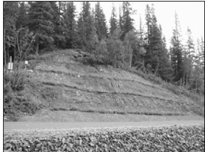
**Fig. 2. New building and upgrade: Soil bioengineering measures to stabilise unsteady slopes (courtesy of Rankka, 2005)/**
