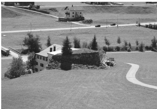
Figure III.2-6. New building and upgrade: Splitting wedge for splitting and deflecting mass movements.
