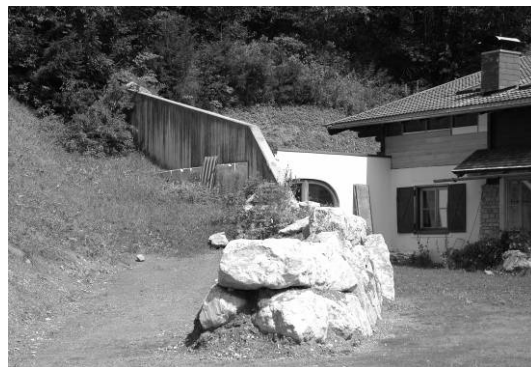
Figure III.2-7. New building and upgrade: Deflection wall.
